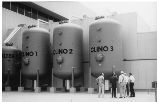
FIG. 4. Clinoptilolite-filled columns at a Denver, CO, water-purification plant [Reproduced with permission from ref. 106 (Copyright 1997, AIMAT)].
